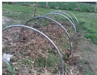
This low tunnel skeleton is constructed from scrap metal that has been cut and bent to the required shape. It was then covered with fabric row cover. Note that soil is used to hold the material against the wind. © Tracy Kittilsen, Dalhousie..
